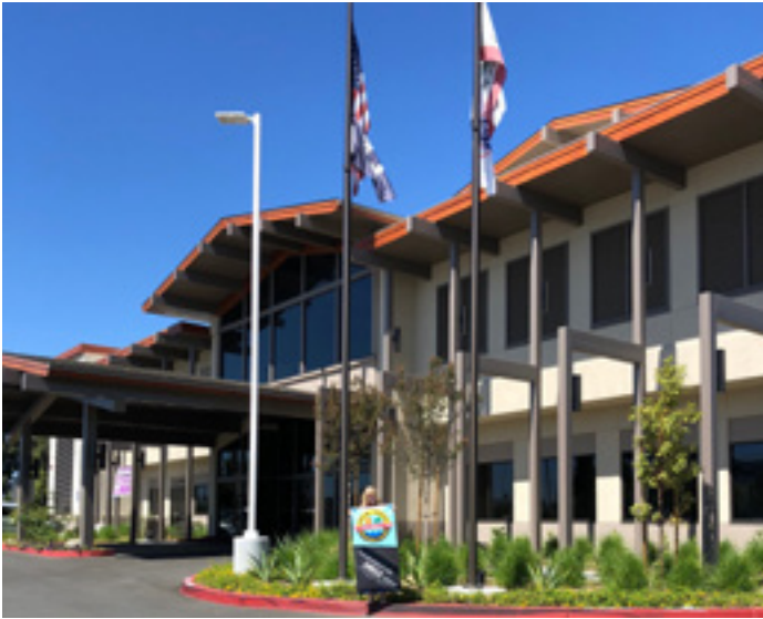
The Elks Lodge in Santa Ana, 55 Fwy and Edinger, 1751 South Lyon Street, Santa Ana, 92705.
