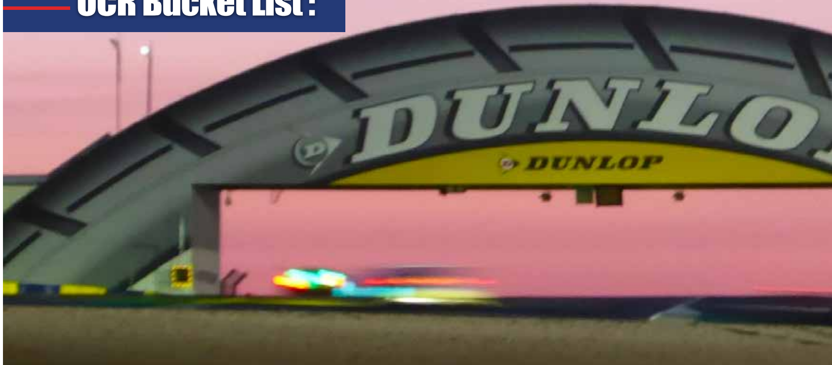
The Le Mans Dunlop Bridge has been there in one form or another since 1932. The 2022 24-Hours of Le Mans is June 11-12. In
